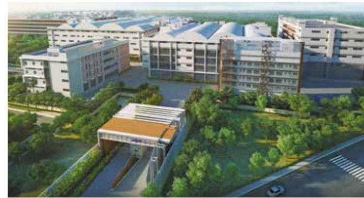
SRIJAN INDUSTRIAL LOGISTIC PARK on NH 6
