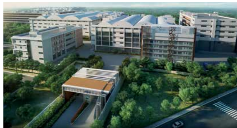
SRIJAN INDUSTRIAL LOGISTIC PARK On NH 6
